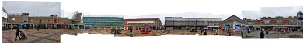
Merseyway South Elevation
