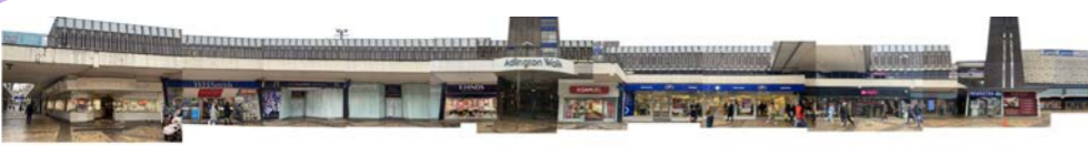
Merseyway North Elevation
