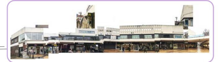
Merseyway North Elevation
