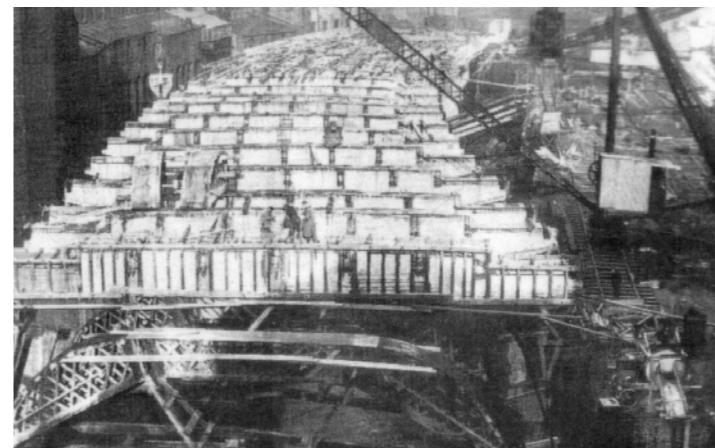
A large stretch of the River Mersey was built over in the 50s to make a highway connecting Bridge Street with Wellington Bridge. Today this is known as Merseyway.
